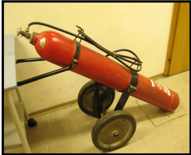
Fig. 19: Transportable fire extinguisher
