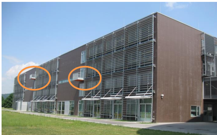
Image 31: The two balconies used to evacuate physically disabled people
