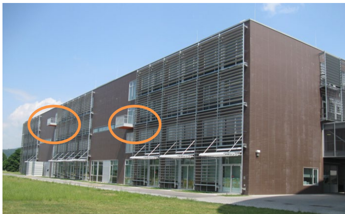
Image 35: The two balconies used to evacuate physically disabled people
